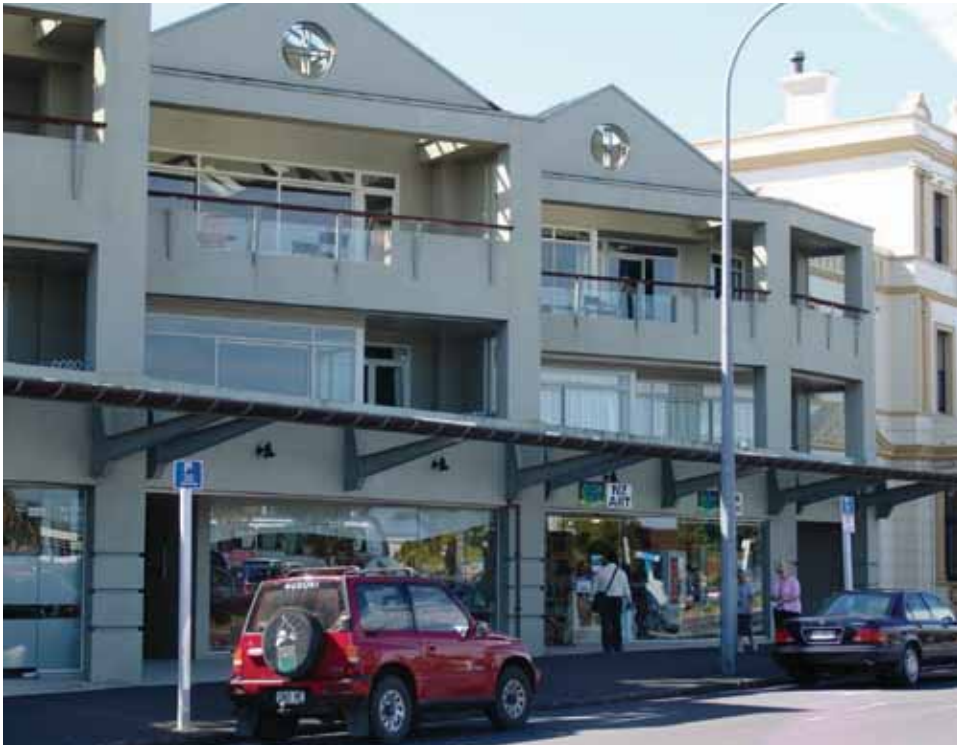
The angled bays provide a strong vertical modulation which reduces the perceived length of the development.
