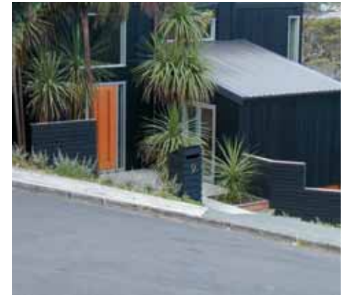
This development has been well designed to follow existing site contours thereby minimising earthworks and soil wastage.
