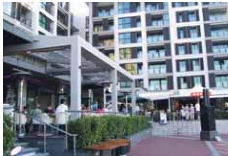
Cafes and restaurants at Viaduct Harbour with apartments above.
