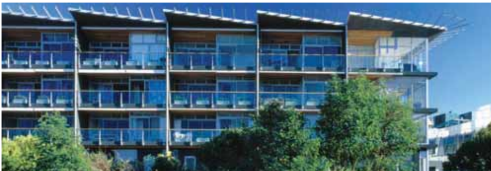
Hemisphere Apartments as viewed from across Augustus Terrace, Parnell.
