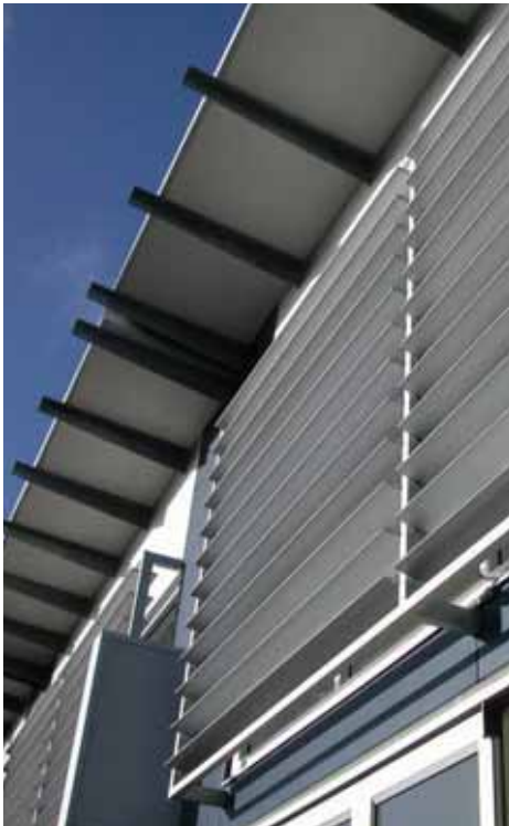
The development utilises passive solar design techniques including external shade devices.
