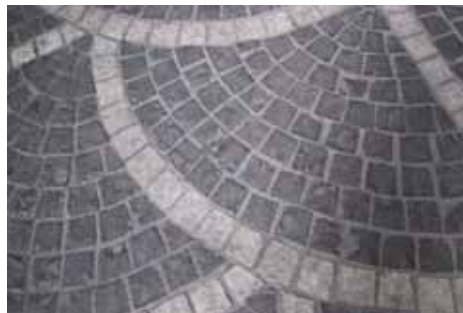
Well-designed paths and walkways are an integral component of landscaping within a development.
