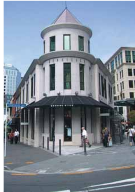
'Wrapping' the corner with façade elements such as awnings or balconies emphasises the building and the corner itself.
