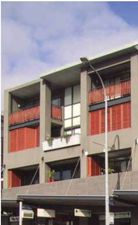
Privacy for residents is maintained by deeply recessing the terraces and providing external shutters.
