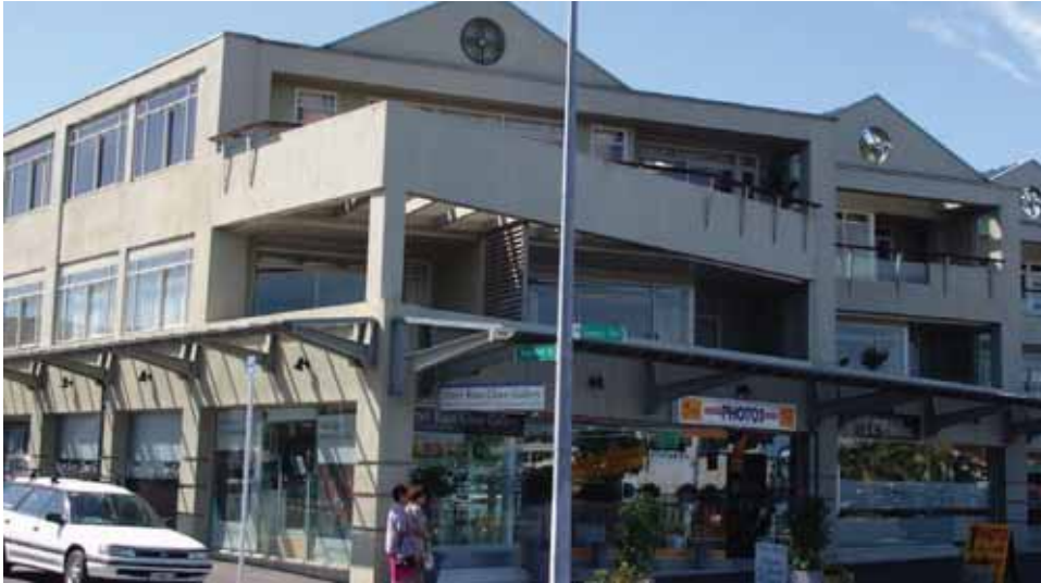
A canopy at ground level and a verandah at first floor level provide design continuity around the street corner.
