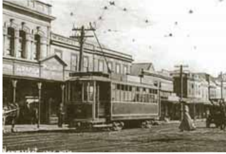
Newmarket in the early 1920s. In many early mixed use buildings shop owners lived above their shops.
