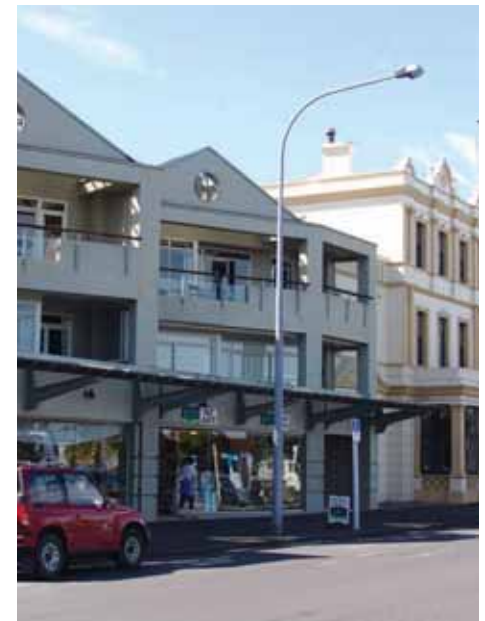
This mixed use development has been designed to integrate with the adjacent historic hotel.
